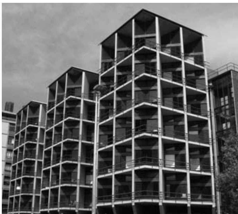
The Erskine building, which houses the Department of Mathematics and Statistics
